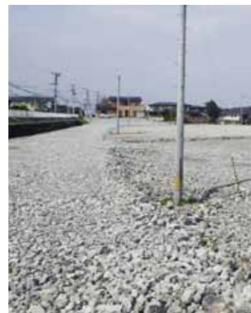
Road using PAMCO Crushed Stone roadbed material
